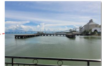
Marine Jetty Lot 2976
